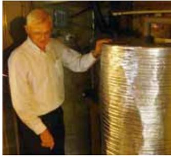
For gas-fired heaters, **make absolutely sure not to cover up the combustion air intake vents at the base of the unit. Also leave a gap a couple of inches wide between the insulation and the flue pipe at the top of a gas or oil heater.**
